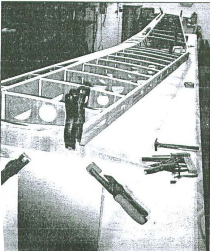
Wing construction finally taking shape. Space to build the 24' wing can be an issue.
